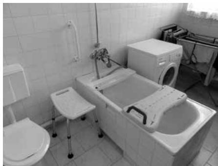
One of the bathrooms for residents at the Social Care Centre in Wieleń
