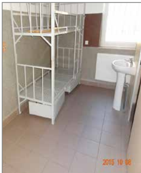
A sink in a cell for persons with disabilities that reduces manoeuvring space, lack of separated shower stalls in the bathroom (Prison in Sieraków Śląski)
