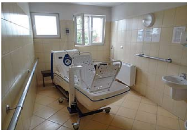
SCH's Elbląg – modern bathroom facilities
