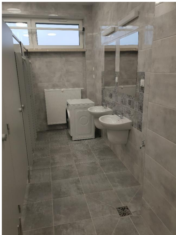
Figure 19. Renovated toilets, GCF in Biała Podlaska.
