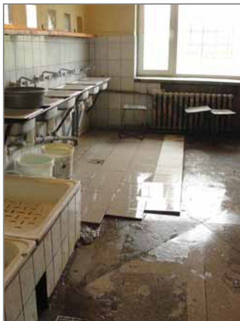
Sanitary facilities in the Prison in Łupków
