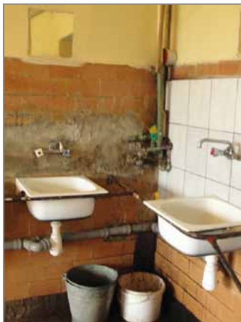
Sanitary facilities in the Prison in Łupków
